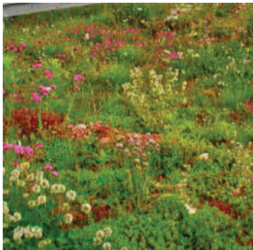
Sedum type extensive green roof (thin substrate)
