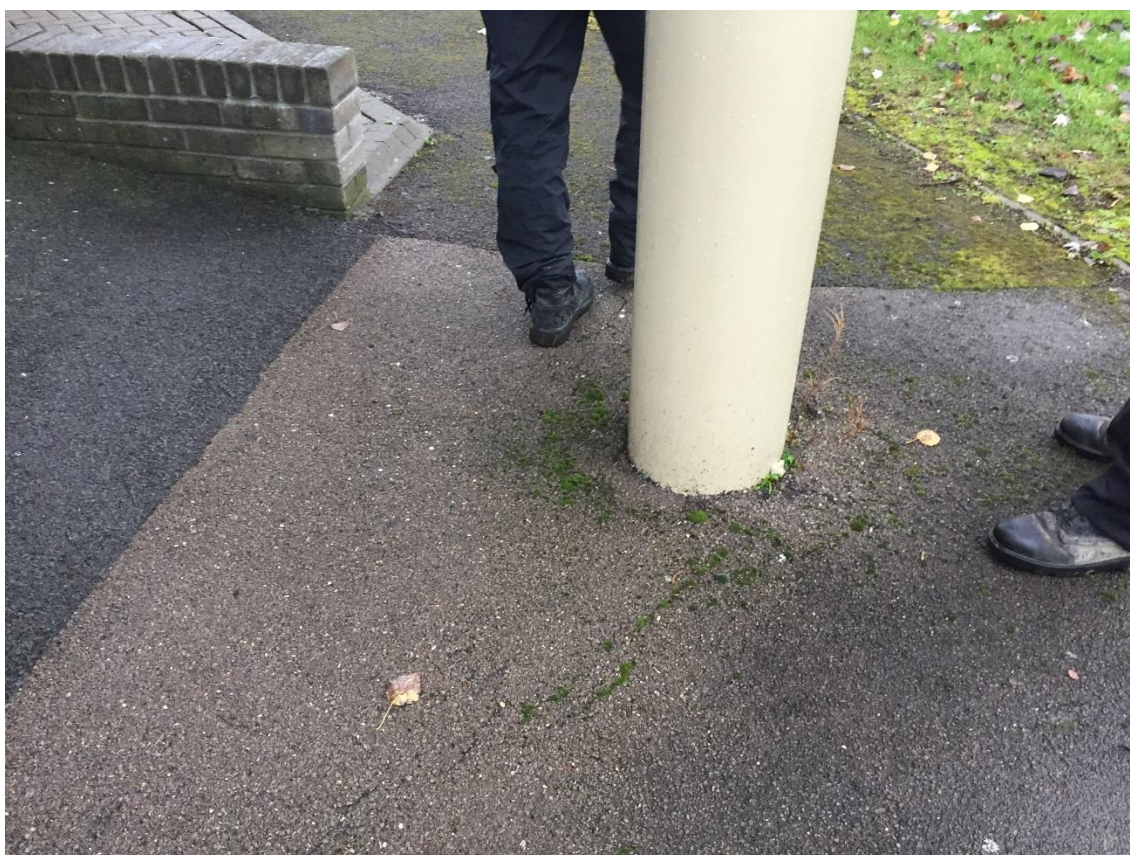
Photograph 14 – Looking at the southern corner of a building in the existing business park. Sign of possible slight settlement in pavement.
